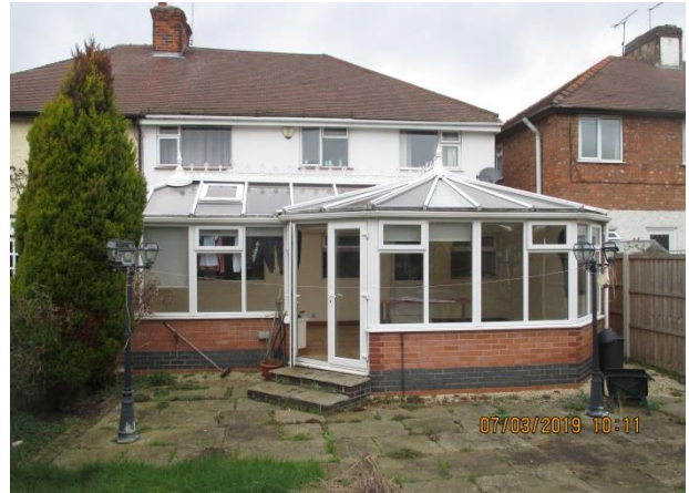
South east (rear) elevation of application property
