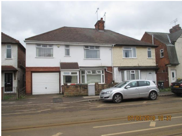
North west (front) elevation of application property
