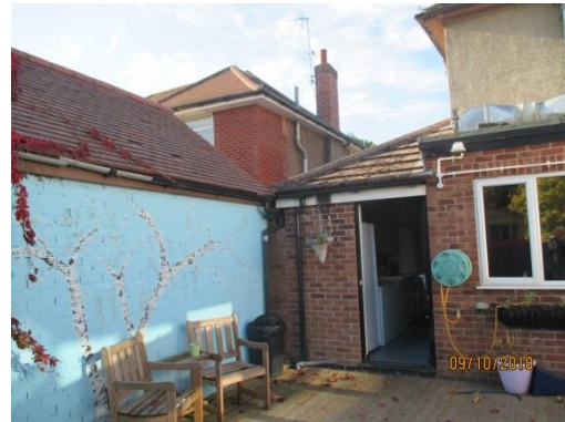
Rear yard, showing garage within 173 Attenborough Lane, forming the south east boundary
